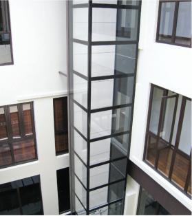
Our most popular product line of screw-driven platform home elevator has a self-supporting shaft enclosure made of panels in steel or laminated safety glass with more than 240 color choices.
